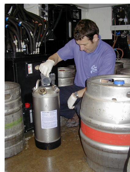
Partially fill the cleaning vessel with water, add the measured amount of P/L PROFESSIONAL and top up with water.
