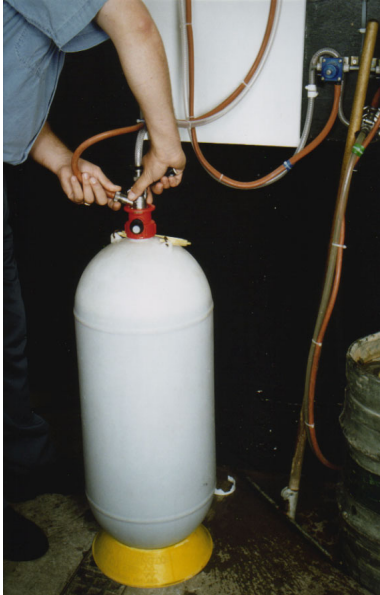
Connect to cleaning ring main
